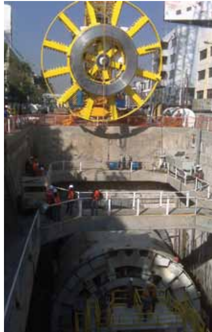
Left: Onsite assembly of major components for the Mexico City Metro's EPB was completed in about eight weeks.
